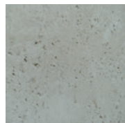
Brut Fort Heavy Pitted
